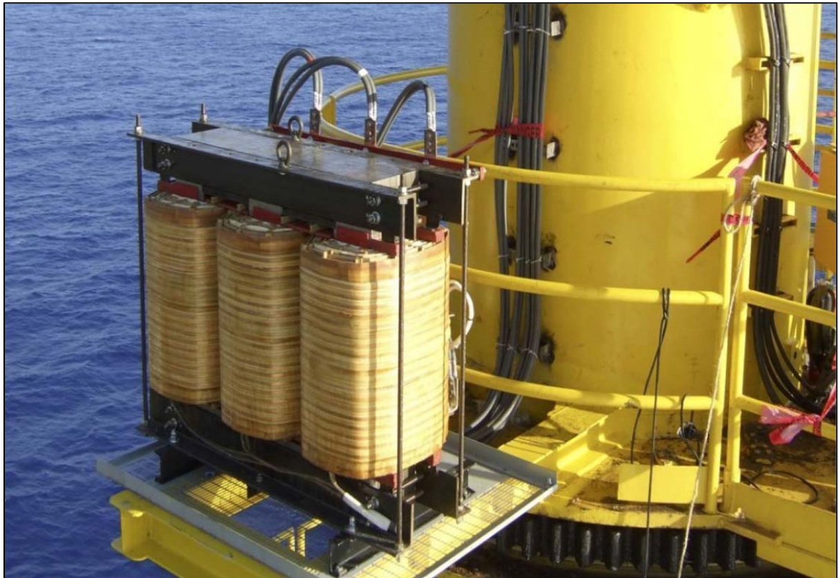
Figure 7.12-6 The new 1MW isolating transformer that cured the CM waveform distortion
