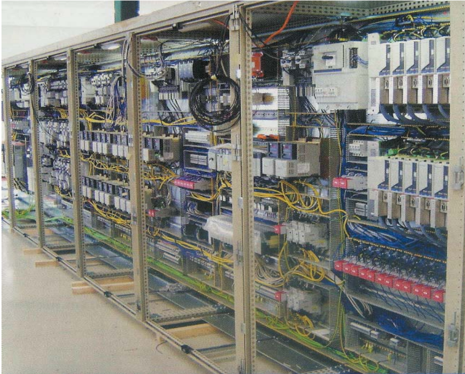
Figure 3: Example of a machine with a number of PDSs Part of a complex installation....
