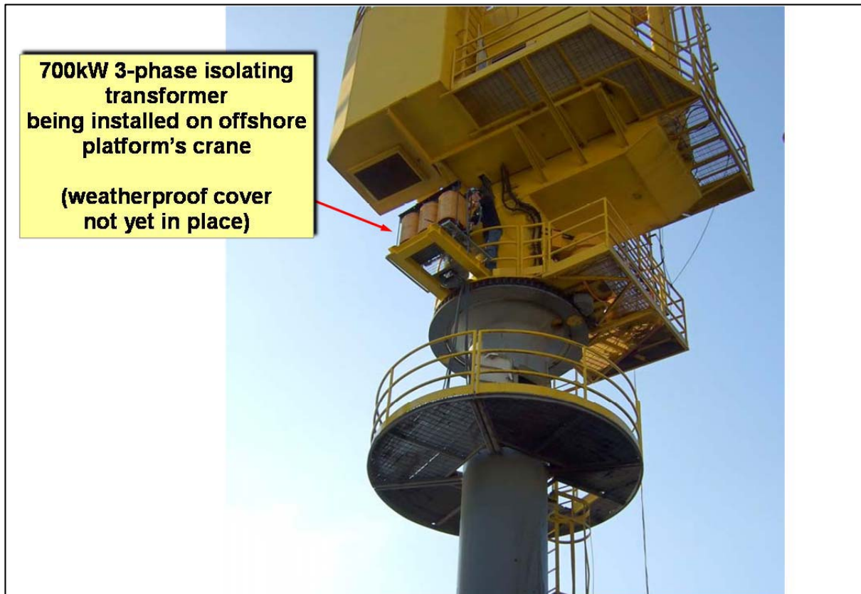
Figure 5.2-3 The fix for the CM noise from the crane motor drives
